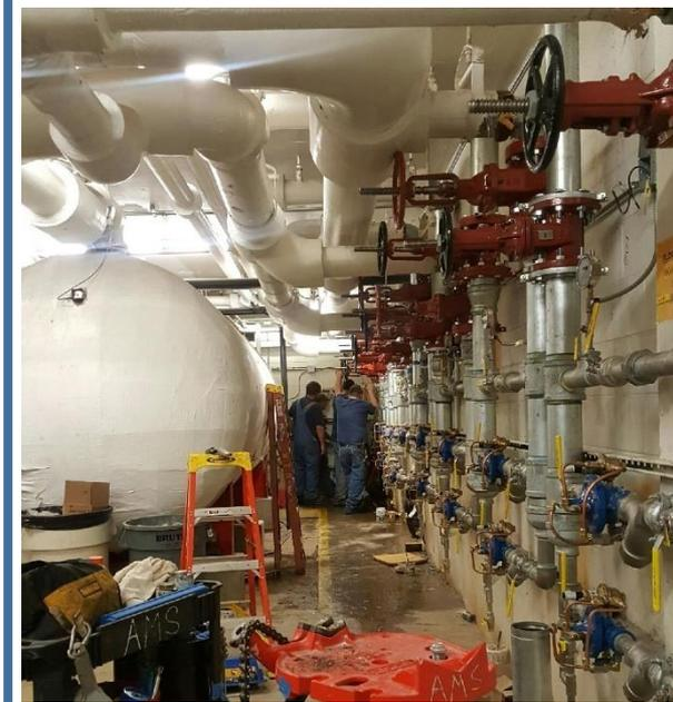
**P4 Level Pump Room with view of the new Cla-Val's (blue devices on wall) and shut off valves above the Cla-Val's.**
